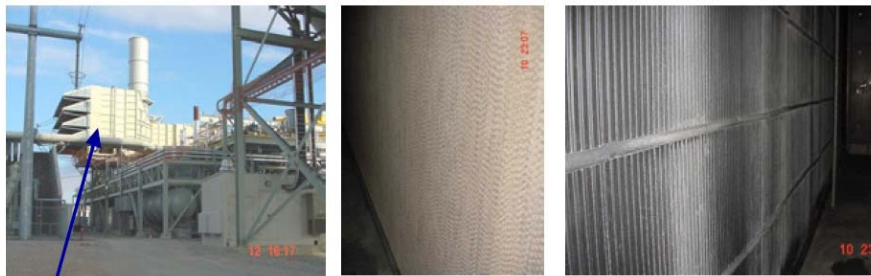
Evap Cooler Location Fig. 57. a) Evaporative Cooler Location, b) Evaporative Cooler, c) Droplet Separator 7
