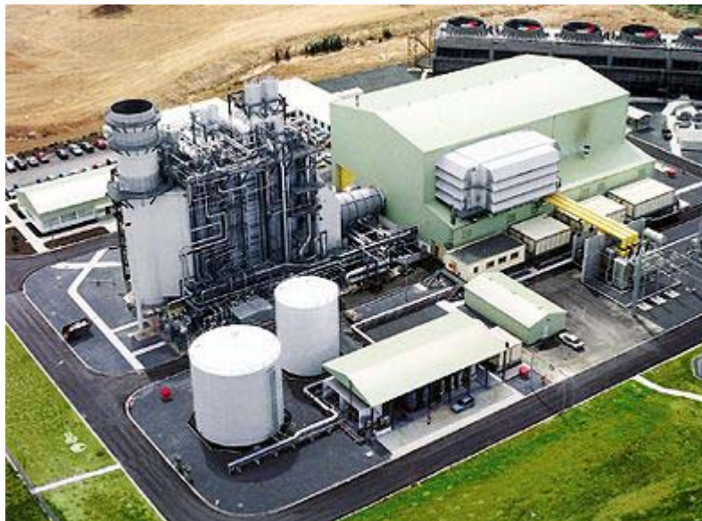
Fig. 74. The 395 MW Combined-Cycle Power Plant Otahuhu, New Zealand uses the modular concept Source: Siemens Westinghouse
