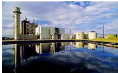
Fig. 7. A simple cycle gas turbine plant, 100 MW simple cycle power plant, Charleston, South Carolina USA, powered by Siemens gas turbines. (Source: Siemens Westinghouse)
