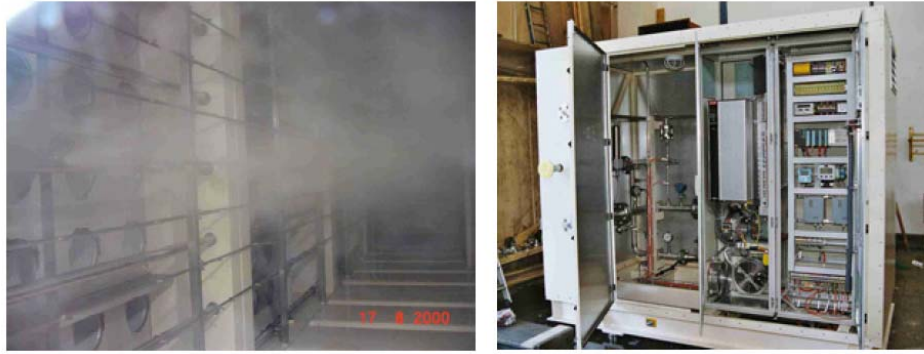
Fig. 59. a) Fogging Nozzle Rack, b) Fogging Pump Skid 7
