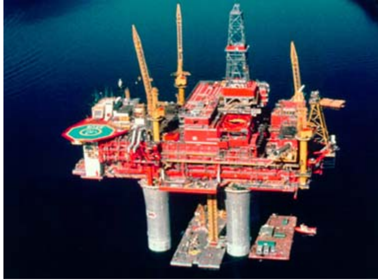
Fig. 10. Gas turbines in offshore service: Offshore platforms produce their own power. Power plant selection is generally an aeroderivative (for weight considerations) gas turbine in simple cycle operation. (Source: GE Power Systems)
